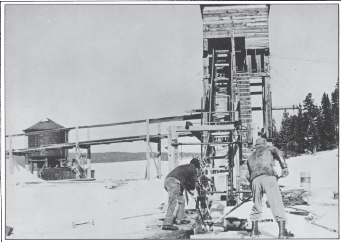
To move ice from the pond to Great Northern Railway cars. Marguerite's crew used a conveyor belt that carried the ice blocks up into a thirty-foot-high tower. The workers loaded five to eight freight cars a day by dropping the ice down a chute from the tower.
