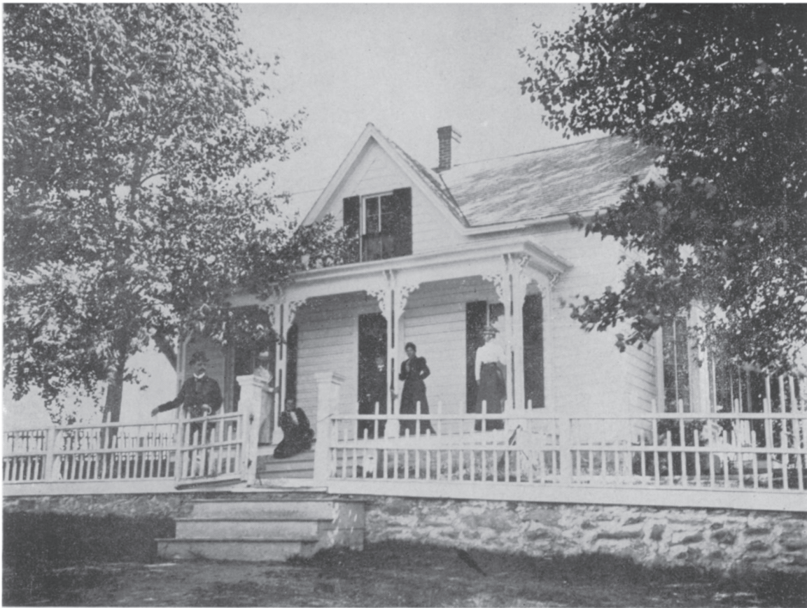
SANDERS HOME in Virginia City, to which Mrs. Sanders was so anxious to return after her tedious journey from the "States" in 1867, is pictured here in 1899 when it was occupied by the family of A. W. Hall. Below is pictured Virginia City's main street at the height of its activity. (Historical Society of Montana photos.)
