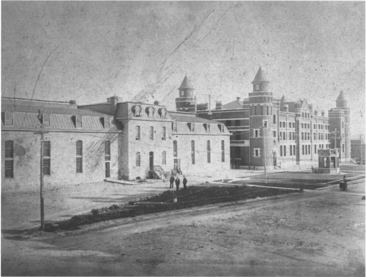
Crude log buildings and the third floor of the territorial prison, the building on the left in this photograph, housed female inmates before the completion of a brick “female department” in the early 1890s. The other building shown is the men’s cellblock built in 1896. A 1959 earthquake damaged the cellblock, and it was torn down the same year; the territorial prison had been demolished in 1931.
