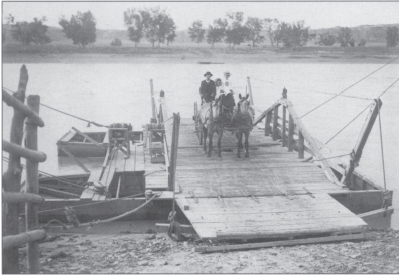
Before 1910 when a bridge was built, cable-drawn ferries like the one above provided the only means for people near Terry to cross the Yellowstone River.
